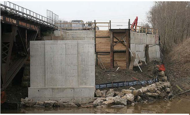
Construction between Port Credit and Oakville
