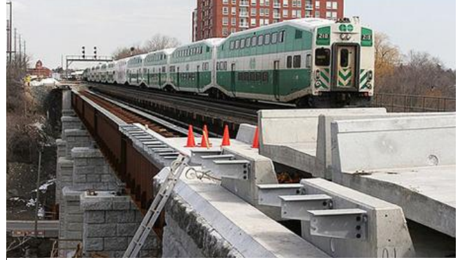
Construction between Port Credit and Oakville
